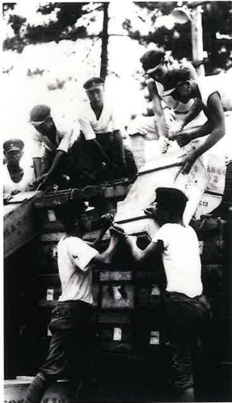
Students working at the Hiroshima Army Depot 1943
