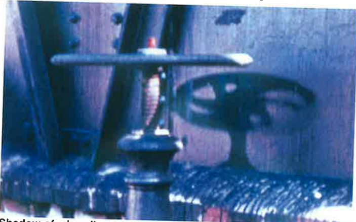
Shadow of a handle on a gas tank Photo by U.S. Army March or April 1946 / 2 km (1.2 miles) from the hypocenter / Hiroshima Gas Co. Hiroshima factory The heat ray burned the coal tar in the paint applied to the surface of the gas tank. The unburned part shielded by the handle retains the original black color.
