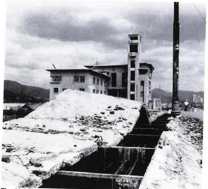
The Aioi Bridge sidewalk lifted Photo by Toshie Kawamoto / Courtesy of Association of Hiroshima A-Bomb Photographers October 1945 / 300 m (328 yards) from the hypocenter
